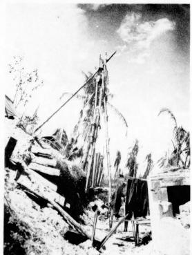
17. Uncompleted section of antitank ditch behind YELLOW Beach showing improvised pile-driver used by Japanese.
