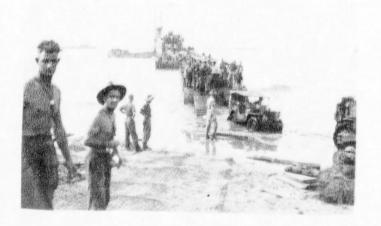
8. LSM unloading vehicles and equipment onto pontoon causeway.
