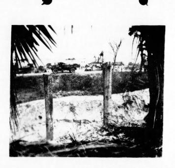
25. Anti-tank ditch from shore side showing spoil bank and log palings.
