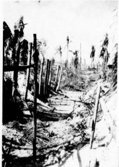
Anti-tank ditch behind YEILOW Beach disclosing placement of log palings.
